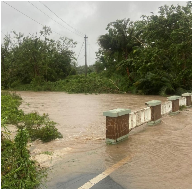
Overflow from the Rio Gurabo covers a road in Puerto Rico following then-Tropical Storm Ernesto on August 14.
