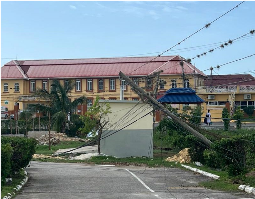
Downed power lines outside a hospital in Saint Elizabeth, Jamaica
