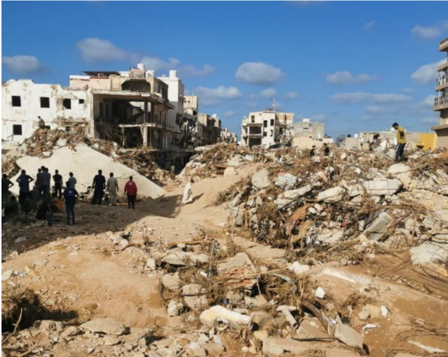
A view of some of the devastation caused by flooding in Derna.
