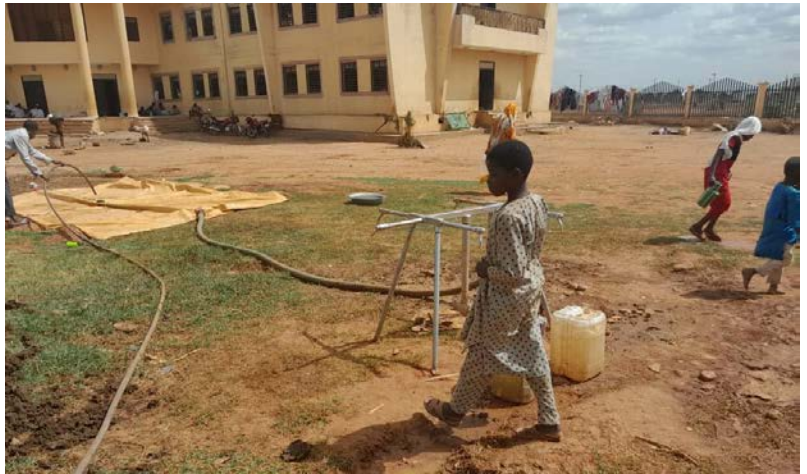
The water supply system in Souqatra IDP camp, Madani, suffered damage after heavy rains, resulting in significant WASH needs.
