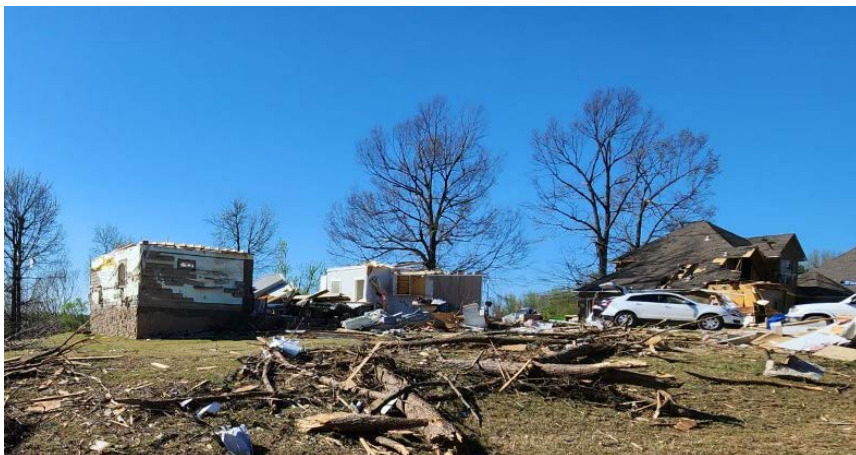
Homes damaged in the wake of the EF-3 tornado that struck Little Rock, AR.
