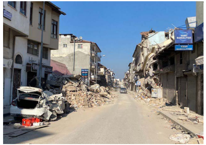
Damage in Antakya, Turkey, the capital of Hatay province, the region hardest hit by the earthquake in Turkey.
