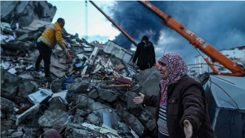
On February 6, a massive 7.8 magnitude earthquake struck Turkey and Syria, leaving tens of thousands dead and injured.
