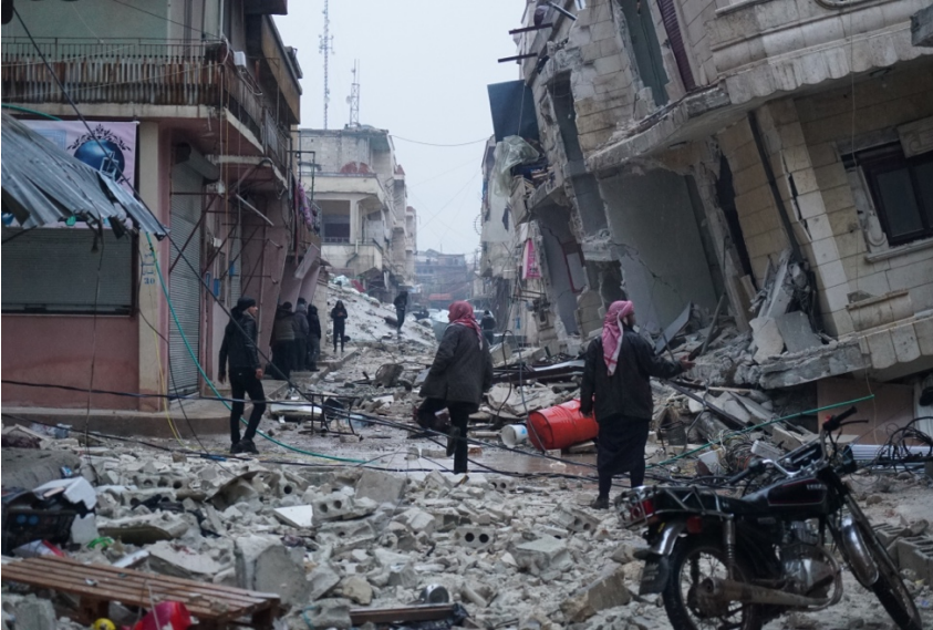
Damage in Jandairis, in the Aleppo governorate in Syria, where dozens of homes and buildings collapsed during Monday's pre-dawn earthquakes. As of February 9, more than 17,000 deaths have been recorded. Source: OCHA
