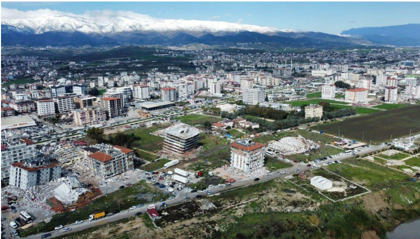
Aerial view of the damage of a residential area in Antakya City in Hatay Province, Turkey, which borders Syria.
