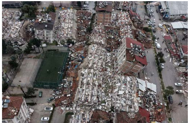
An aerial view of damage to residential buildings in Hatay province, Turkey.
