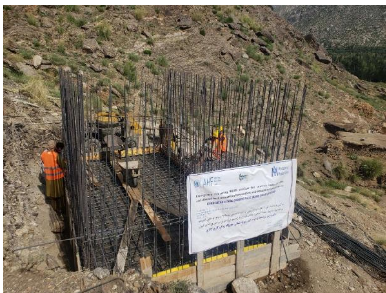
A pipe system under construction in Watapor district of Kunar province.
