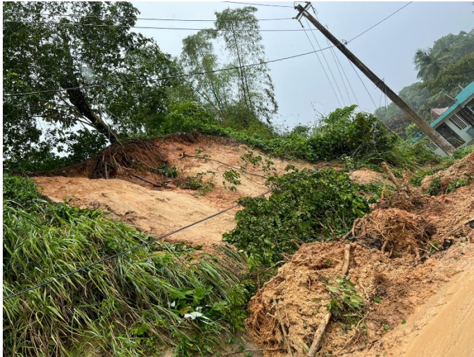
A landslide caused by Hurricane Fiona in the town of Utuado, Puerto Rico.
