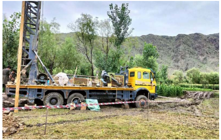
A pipe system under construction in Nurgal district, Kunar province.
