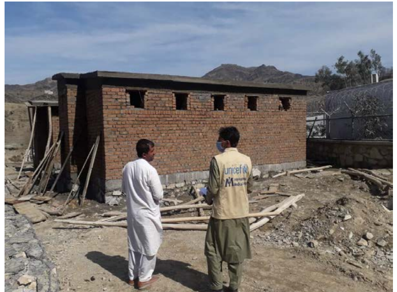
Construction of latrines in Torkham, Durand Line, bordering Pakistan.
