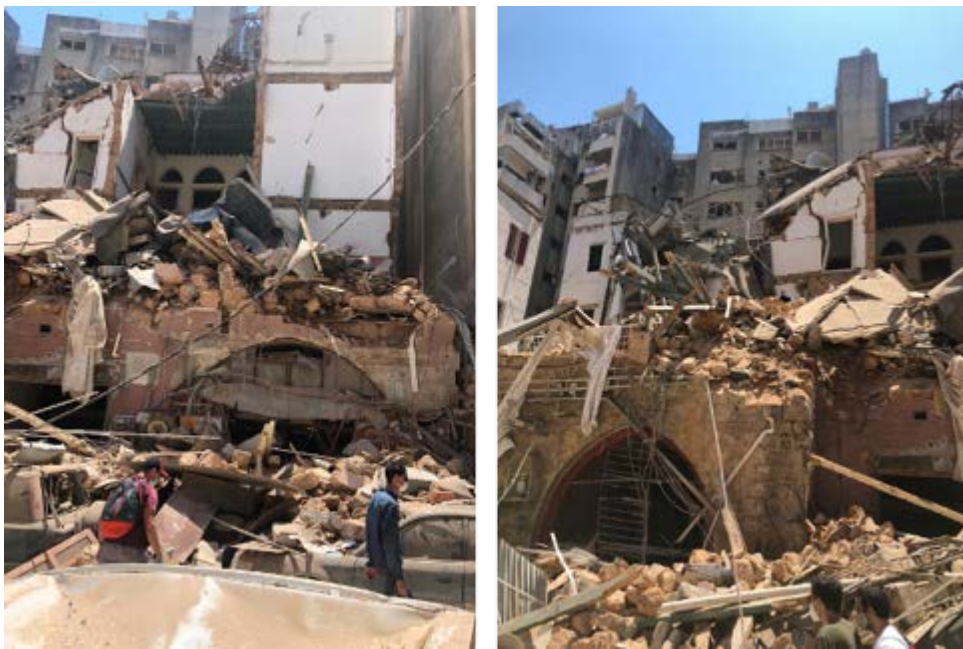
At least 220 people were killed and more than 6,000 were wounded following explosions that erupted in Beirut on August 4. Broken glass and debris could be seen as far as two miles away, encompassing an area where more than 750,000 people live.
