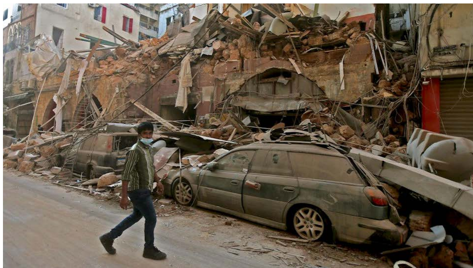
The August 4 explosion in Beirut caused widespread damage, leaving hundreds dead, thousands injured and hundreds of thousands homeless. Photo credit: Wall Street Journal / Agence France-Presse
