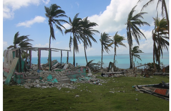
A building in southwest Haiti is reduced to rubble by Hurricane Matthew.
